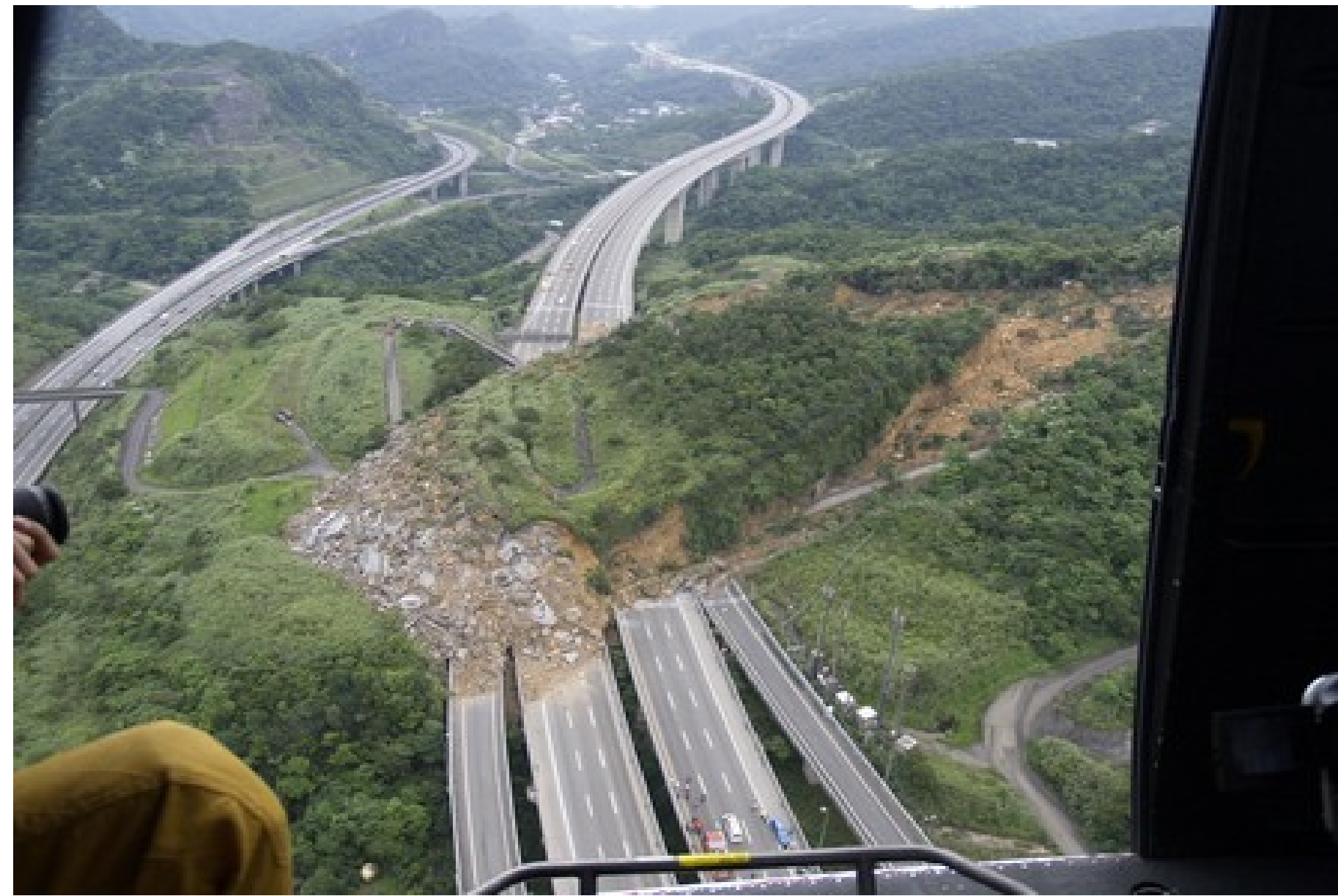
Fig 1: A Landslide at the No. 3 Freeway between Taipei and Keelung, Taiwan 1 .
